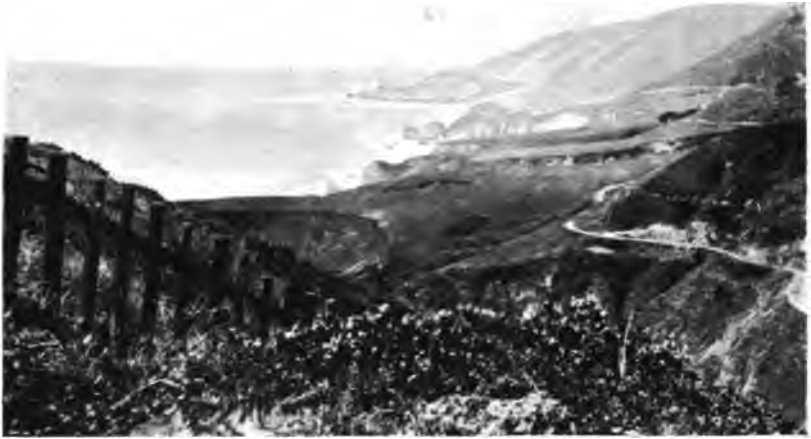
The Monterey Coast south of Carmel showing present road.
